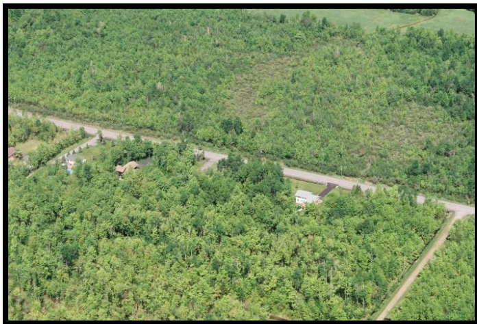
The Limoges Wellhead
