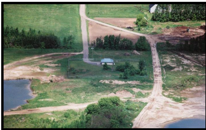
Embrun Drinking Water System
